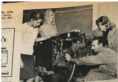
SPARK PLUGS? —Janice Kroesen, Judith Plennmons, Judith Tonini listen to instructor Norman Gibbs explain the purpose of spark plugs and watch him remove them for cleaning and adjusting.
